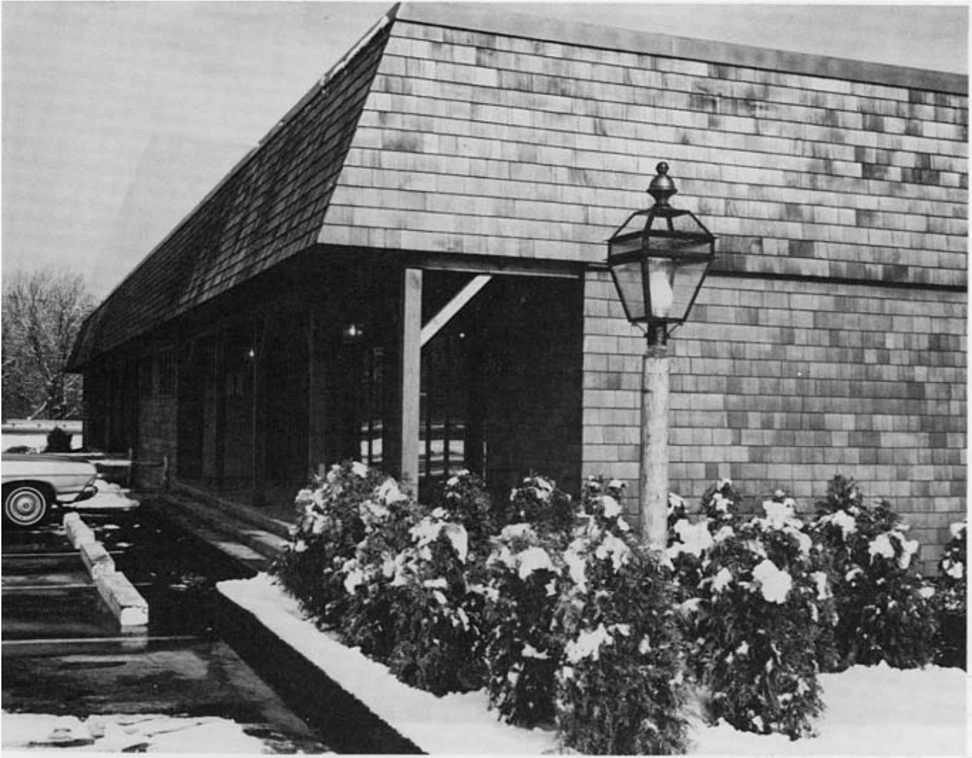
Figure 27 — Application of wood shingles to a commercial structure. (Photo courtesy of the Red Cedar Shingle and Handsplit Shake Bureau)
