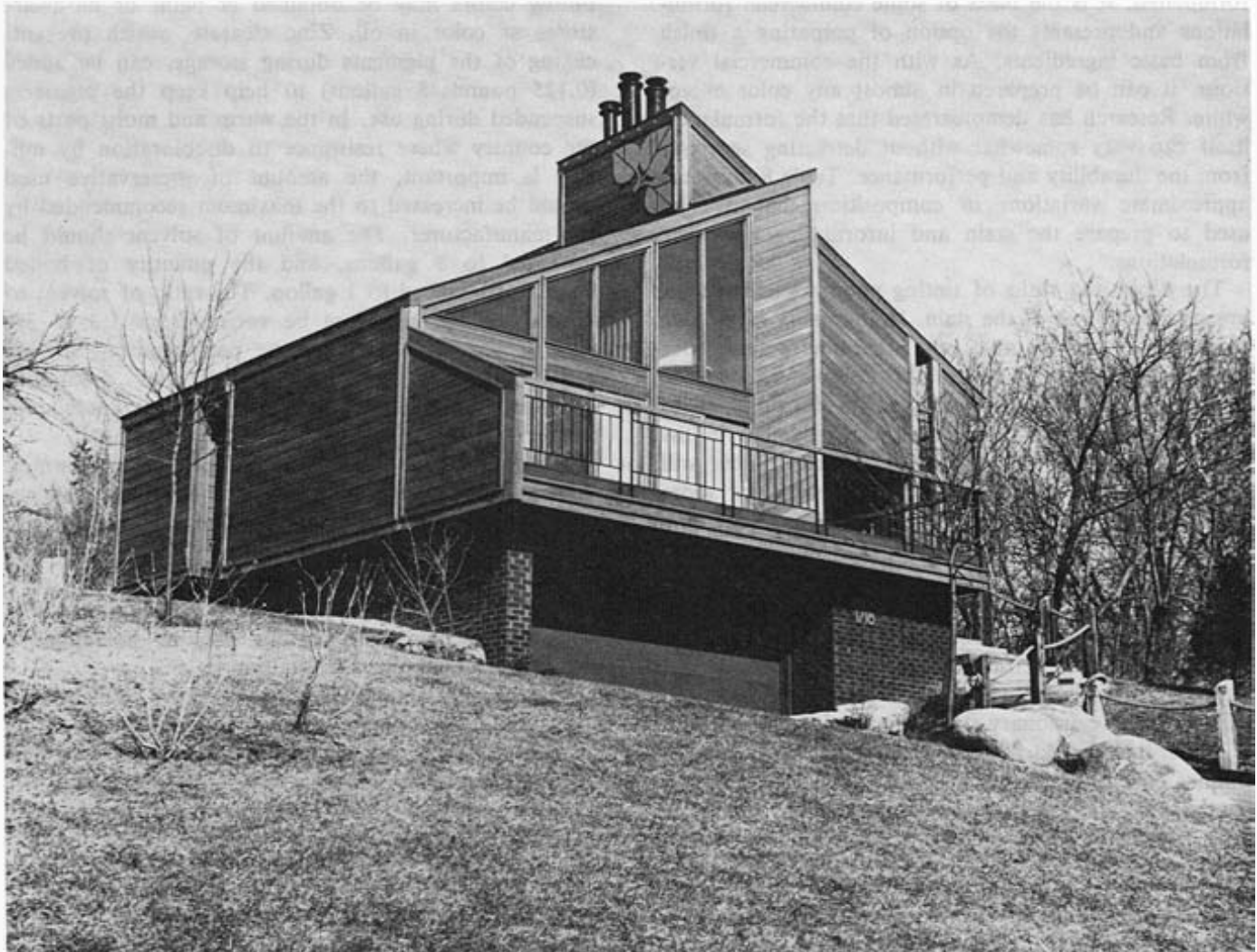
Figure 24 —Modern house finished with a semitransparent penetrating oil-based stain.
