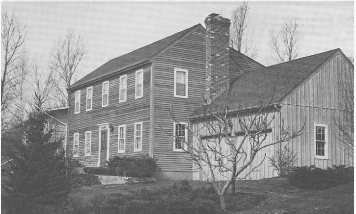
Figure 17 —House with western redcedar siding that has been allowed to weather naturally.
