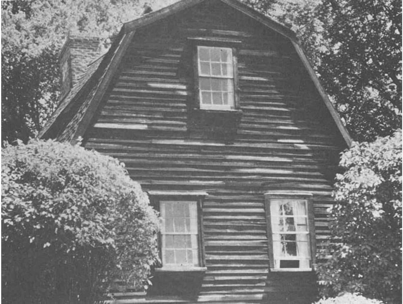
Figure 14 —Old Fairbanks house at Dedham, Massachusetts built in 1637. Most of the white pine clapboard siding was replaced in 1903 and has stood 80 years without paint.
