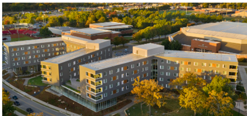
Figure 2. Adohi Hall, University of Arkansas campus, Fayetteville, AR (MODUS Studio).
