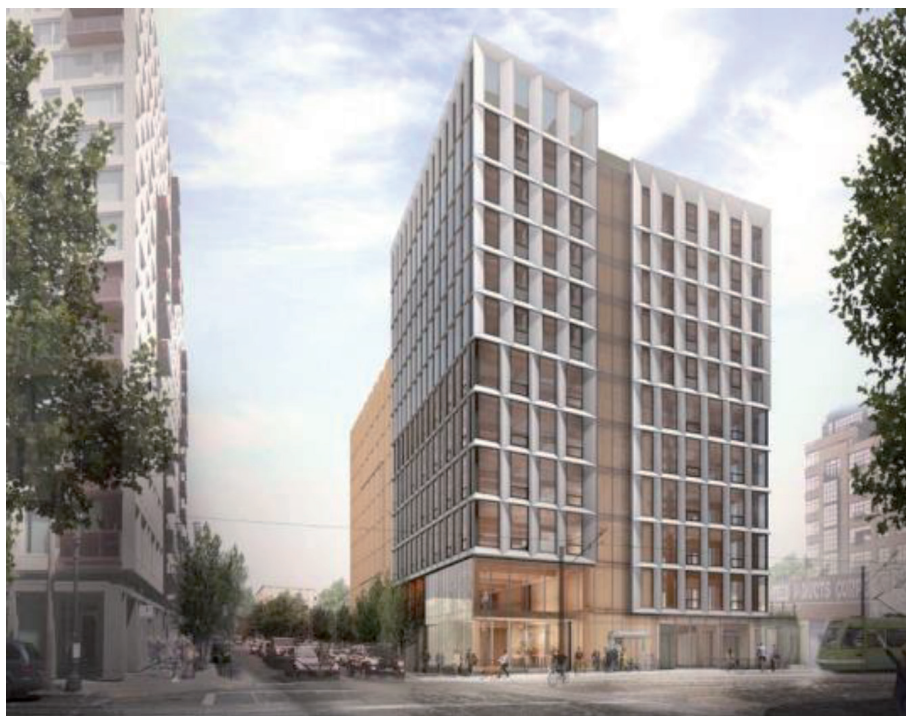
Figure 1. 12-story framework building with mass timber from ground floor (not built) designed for Portland Oregon US (Credit: Lever Architecture).
