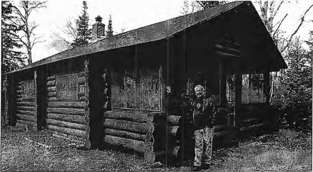
Figure 10 - Completed rehabilitation to the U.S. Forest Service Bearskin log cabin in October 2009.
