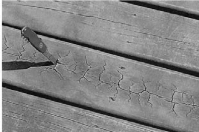
**FIGURE 7.5** Cross-grain checking in juvenile wood.
