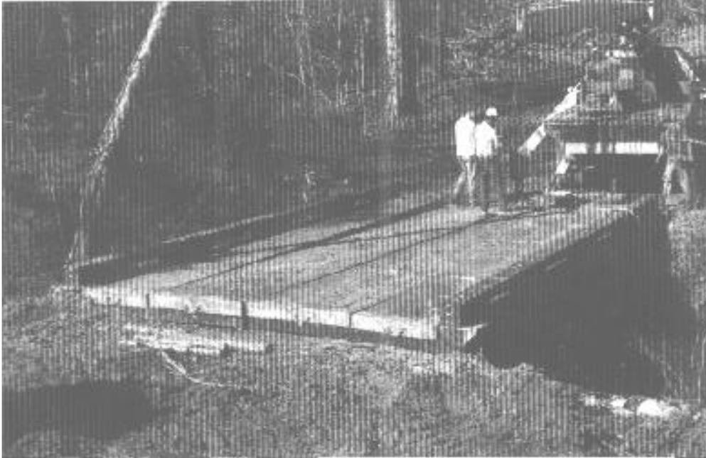
Figure 1. Portable longitudinal glulam deck bridge for truck traffic.
