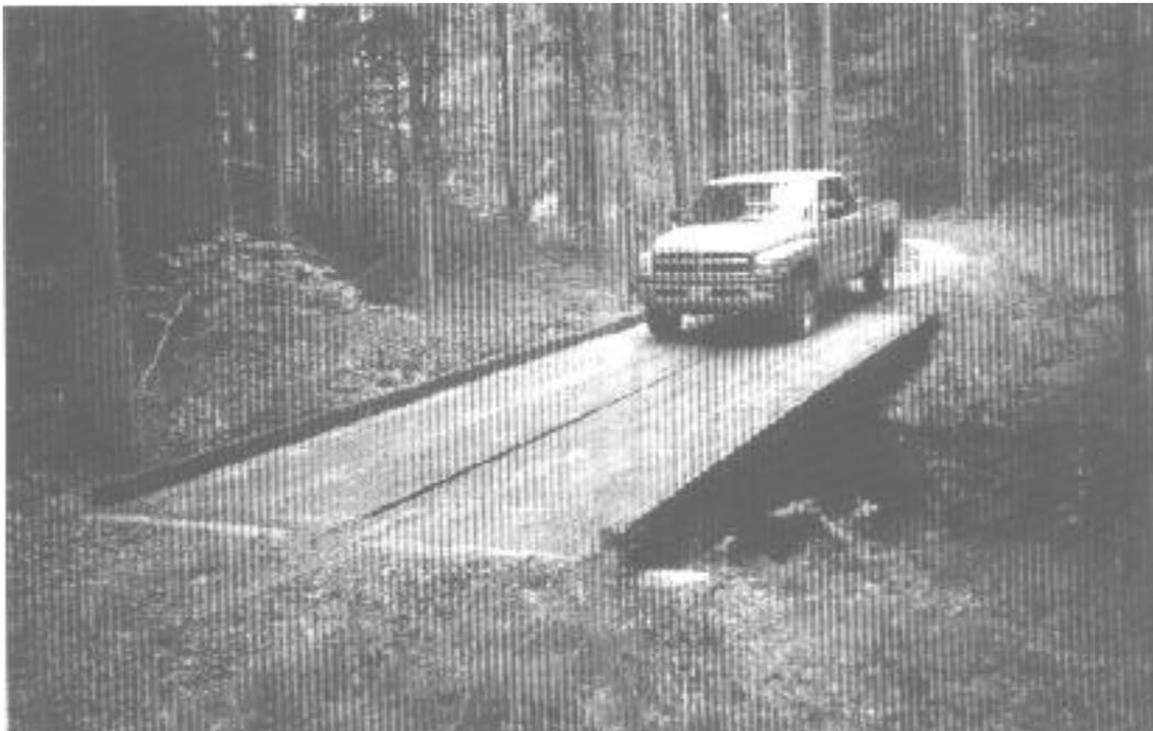
Figure 3. Portable T-section longitudinal glulam deck bridge.
