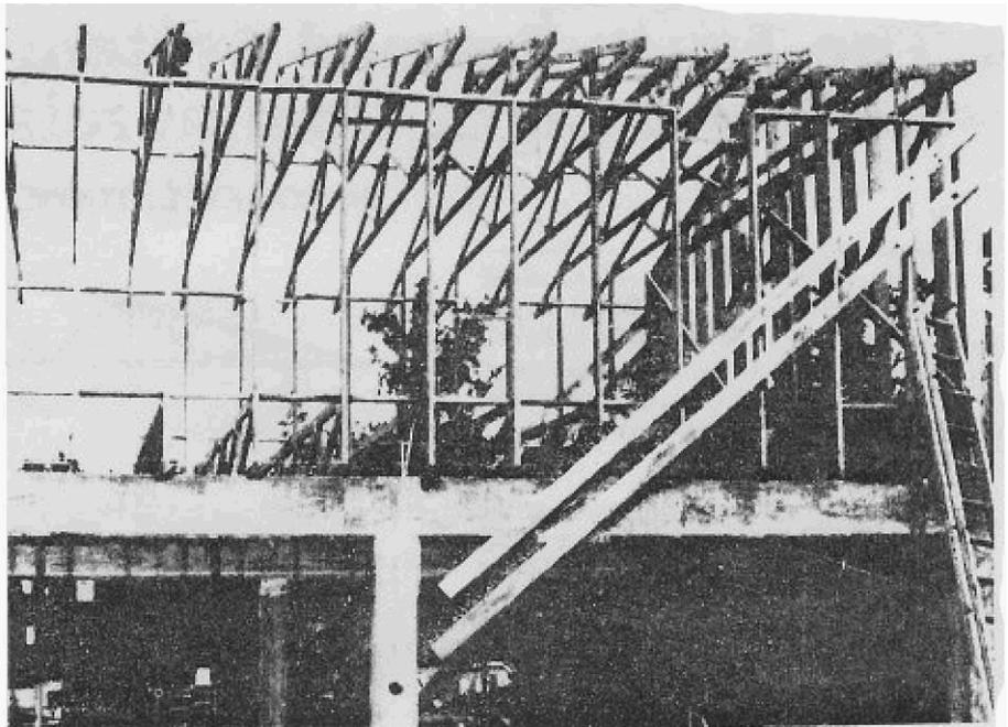
*FAST—Florida Keys Truss, Inc., recently erected a 1500 square foot house in two hours and 50 minutes. It was built on an elevated concrete beam and pedestal foundation for protection from storm surge during hurricanes (Photo—Florida Keys Truss, Inc.)*
