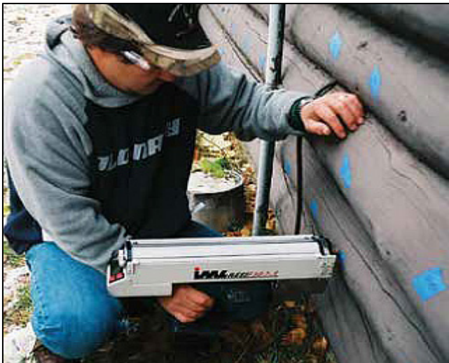
Figure 10—A resistance microdrill being used for inspection of a historic Civilian Conservation Corps log cabin.
