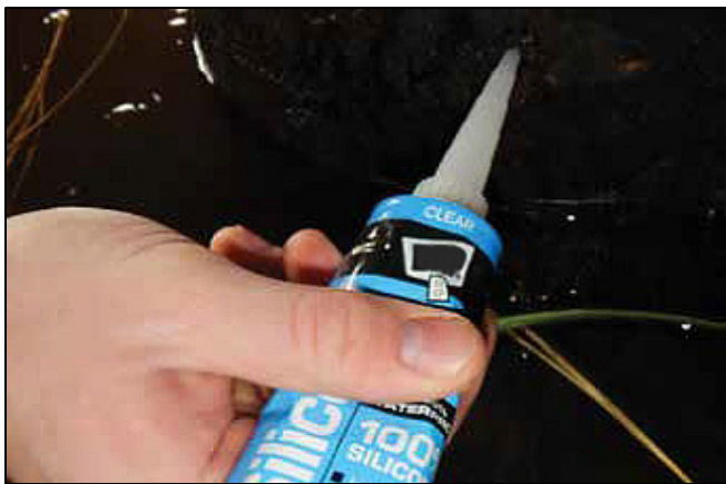
Figure 15—Silicone is used to fill the small drilling hole.
